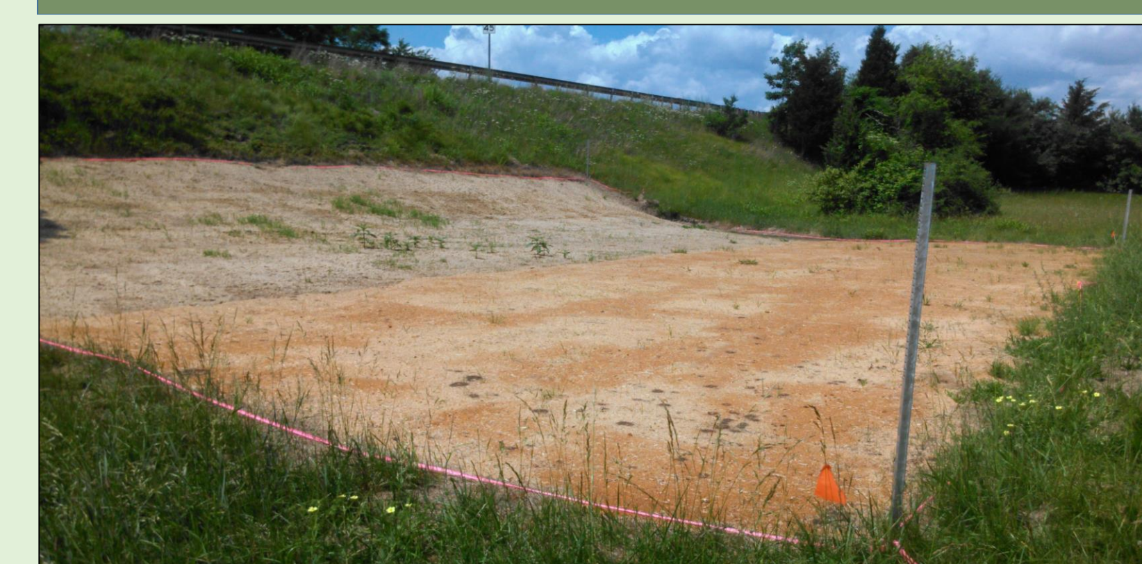
A site along Rte. 6 planted using sawdust
